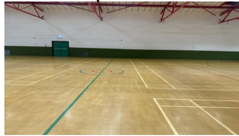
Picture 2 – Sports Hall Side Wall
