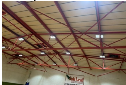
Picture 3 – Sports Hall Roof Steel Work
