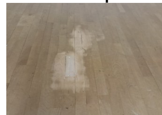
Picture 4 – Squash Court Flooring Minor Repair
